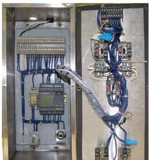
Tru-flo control wiring schematic and photo with SC supply control Figure 19
